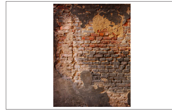
F04: EXPOSED BRICK WALL
