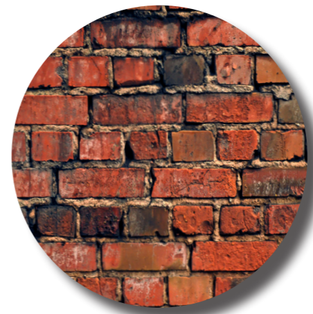
EXPOSE BRICK IN AREA A3
